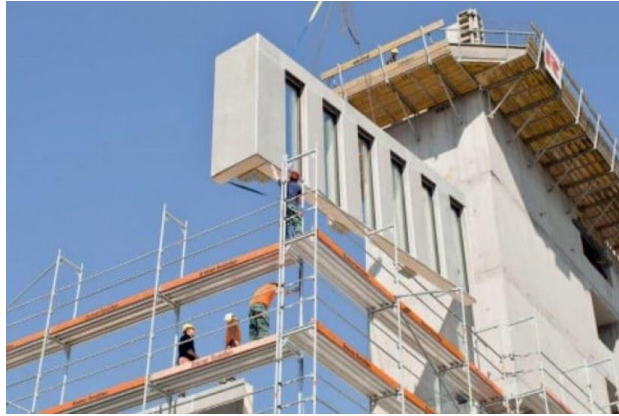
(Fig. 32 Hybrid Concrete Construction)
