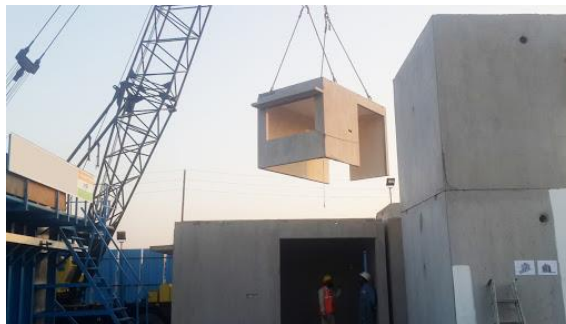
(Fig. 31 3D Volumetric Construction)
