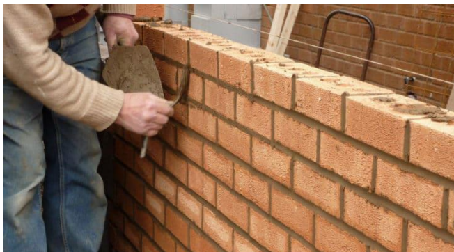
(Fig. 36 Thin Joint Masonry)
