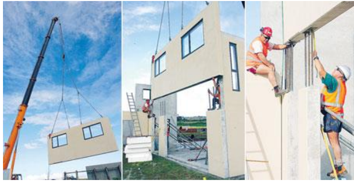
(Fig. 34 Precast Flat Panel System)
