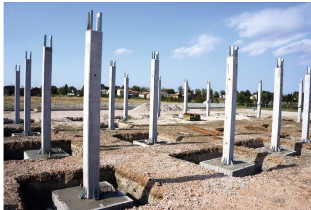
(Fig. 35 Precast Foundations)
