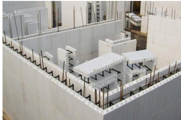
(Fig. 33 Insulating Concrete Formwork)
